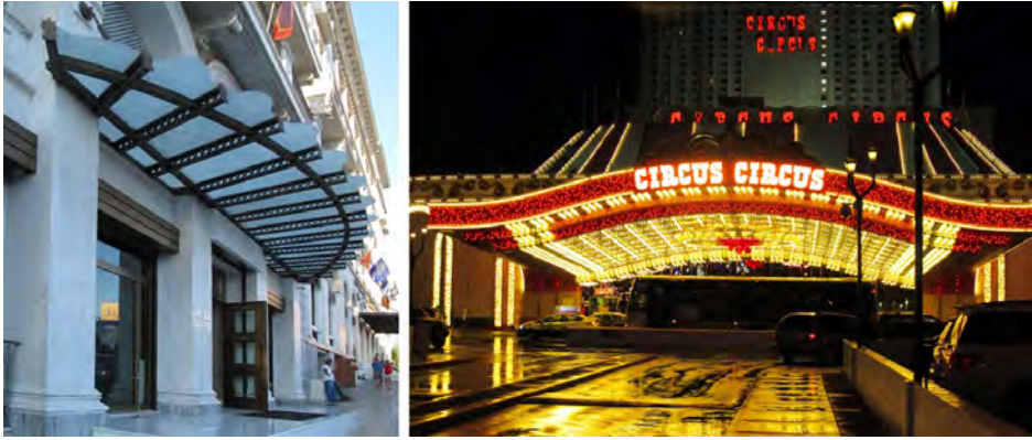
Fig. 2. Roofing over the main entrance – two extreme solutions. First: gentle decorative, glassed element in NJV Athens Plaza in Athens (Greece). Second: large-scale light and commercial element of Circus Circus in Las Vegas (Nevada, USA)
