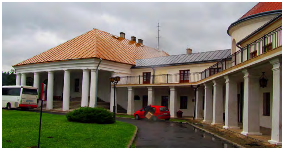
Fig. 1. The representational and hospitality transition zone between exterior and interior in the historic castle in Lesko, Poland (building started in the XVI century), which served both as residence and accommodation zone for guests
